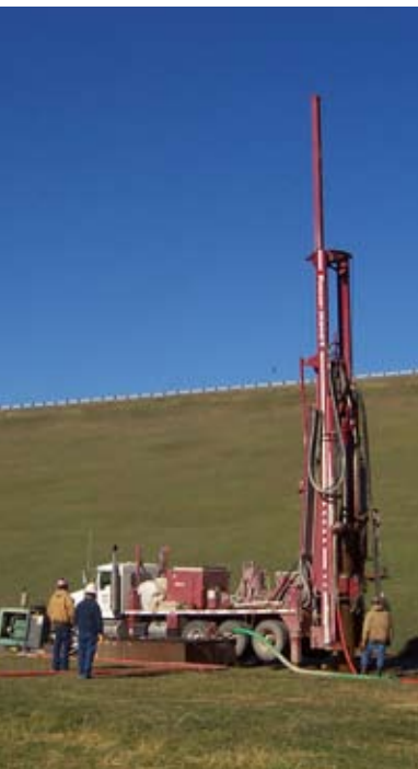
WORKERS DRILL FOR NEW RELIEF WELLS AT ENGLEWOOD DAM.
